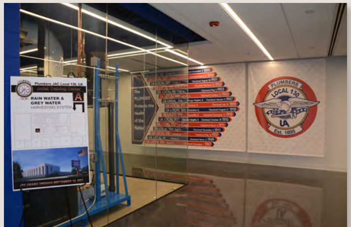
Rain Water and Grey Water Harvesting Systems.
